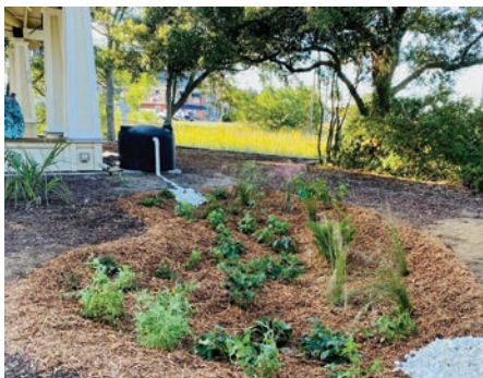
Rain Gardens with Cistern
