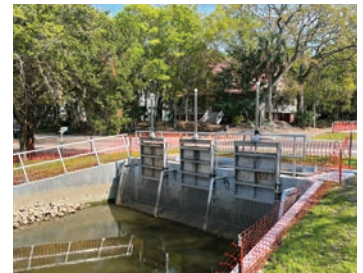
Improved drainage structure
