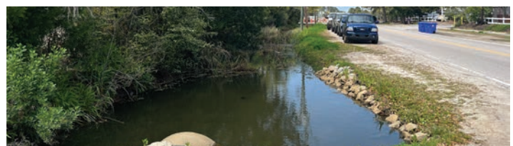
Cleaned and reinforced existing ditch in the right-of-way
