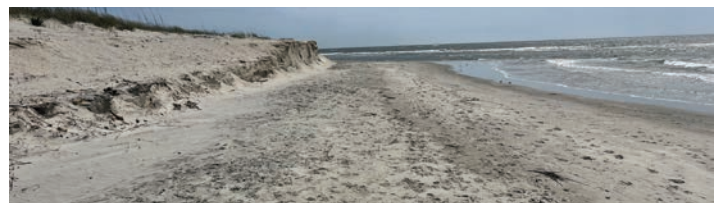
Beach nourishment at Breach Inlet
