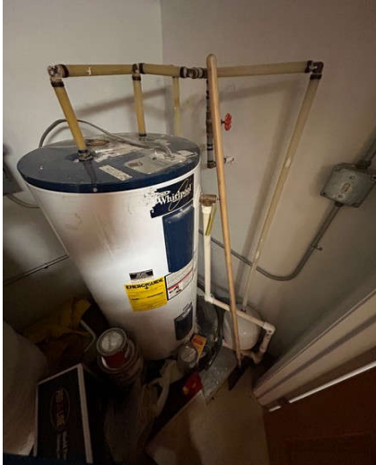
2 nd Floor Sink @ Conf Room
