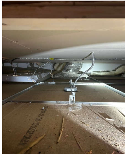
2 nd Floor Above Ceiling/Sub-Ceiling
