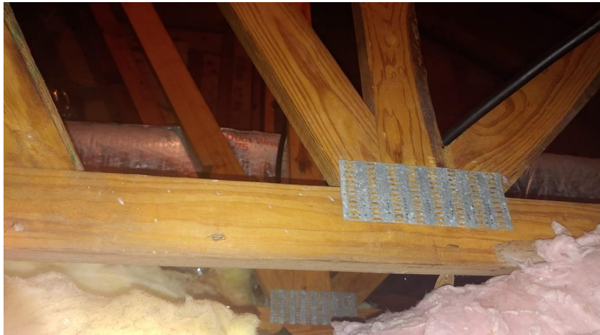
Photograph No. 2 Roof Framing: Metal Plate Connected Wood Trusses
