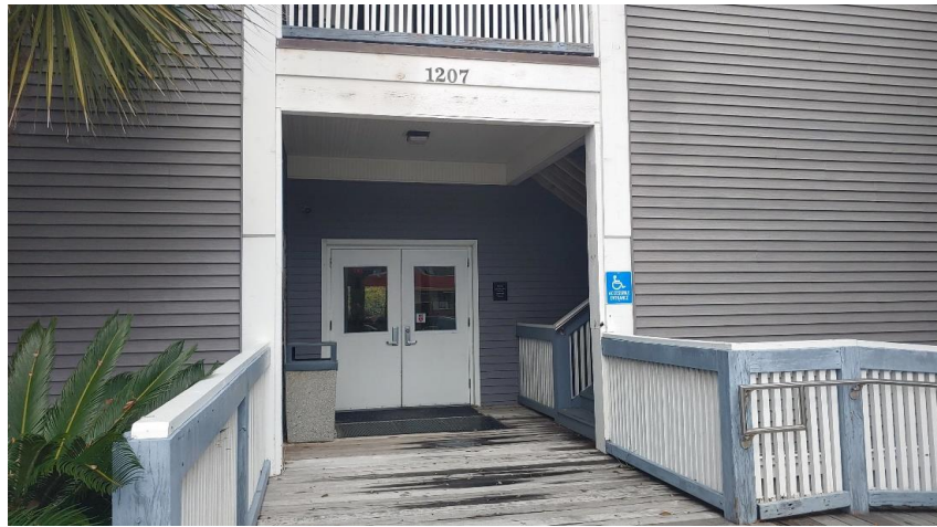
Photograph No. 13 Front Entrance
