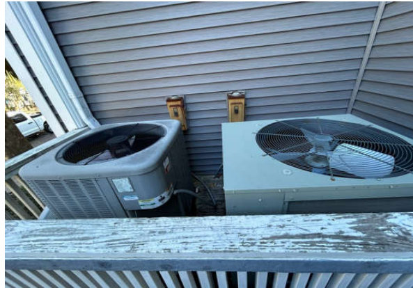
West Side CU Platform
