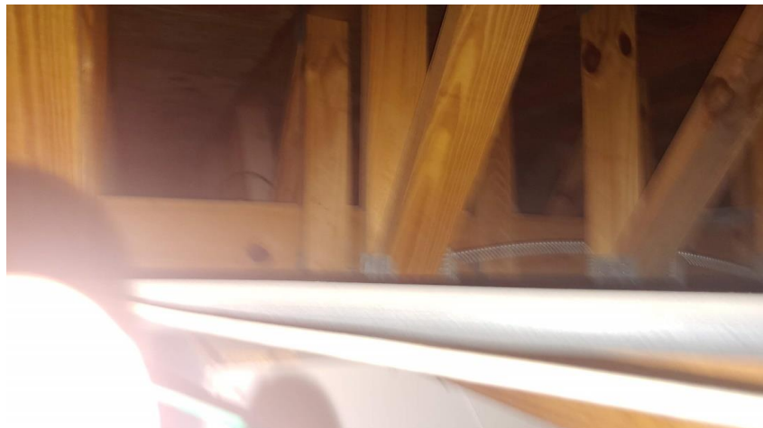
Photograph No. 8 Second Floor Framing: Metal Plate Connected Wood Trusses
