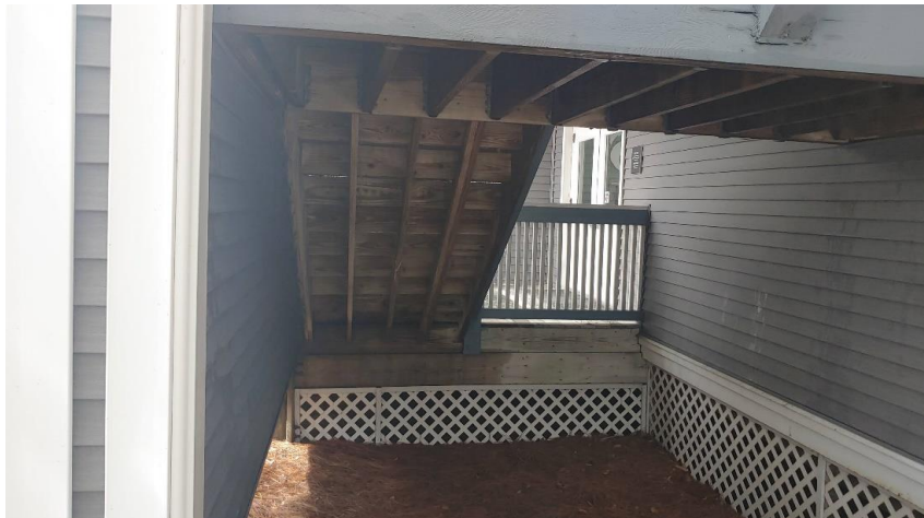
Photograph No. 18 Front Entrance, Stair and Landing Framing
