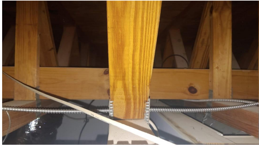
Photograph No. 7 Second Floor Framing: Metal Plate Connected Wood Trusses
