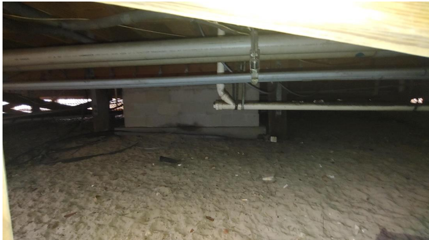
Photograph No. 10 First Floor Framing: CMU on Pile Cap at Elevator
