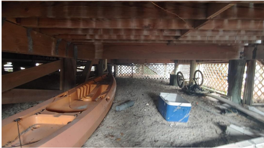
Photograph No. 9 First Floor Framing: Joists, Beams, Piles
