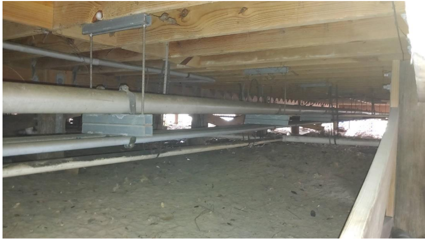
Photograph No. 11 First Floor Framing: Joists
