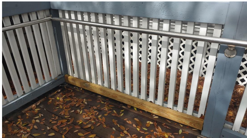
Photograph No. 16 Guardrail at First Floor Level, Repairs in progress
