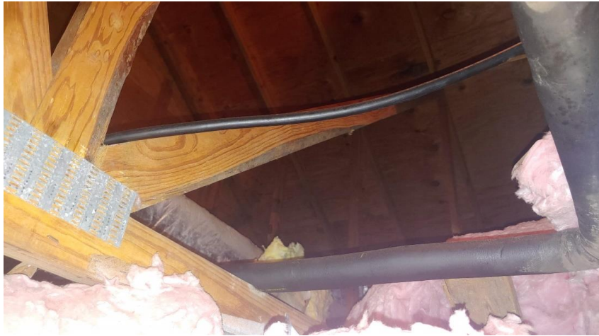
Photograph No. 1 Roof Framing: Metal Plate Connected Wood Trusses
