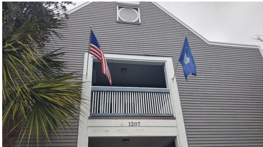
Photograph No. 14 Front Entrance
