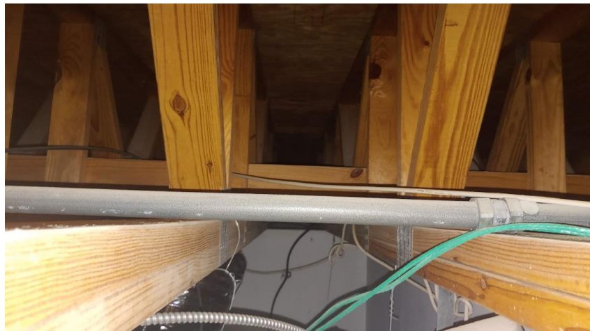
Photograph No. 6 Second Floor Framing: Metal Plate Connected Wood Trusses
