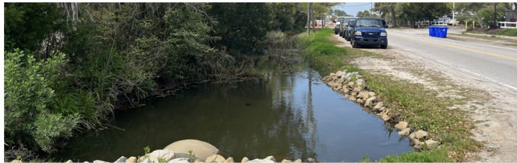
Cleaned and reinforced existing ditch in the right-of-way
