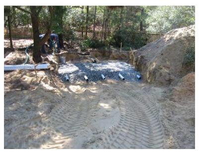
Figure 7-3. Septic system replacement
