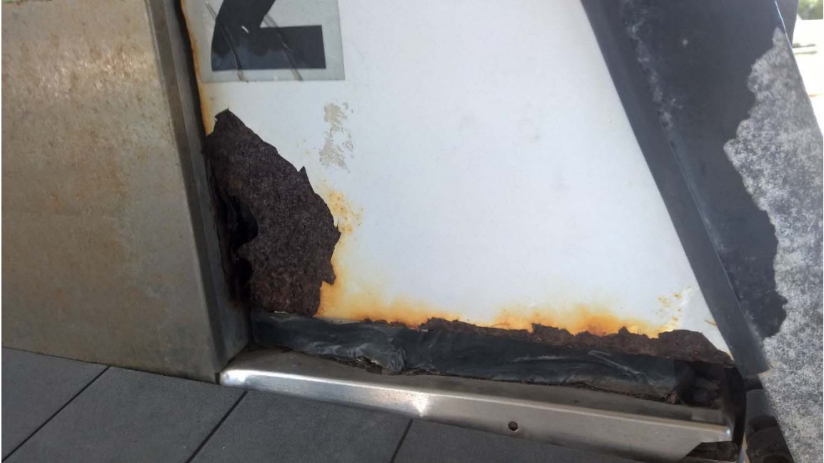
Corroded Fuel Dispenser - Beyond Repair
