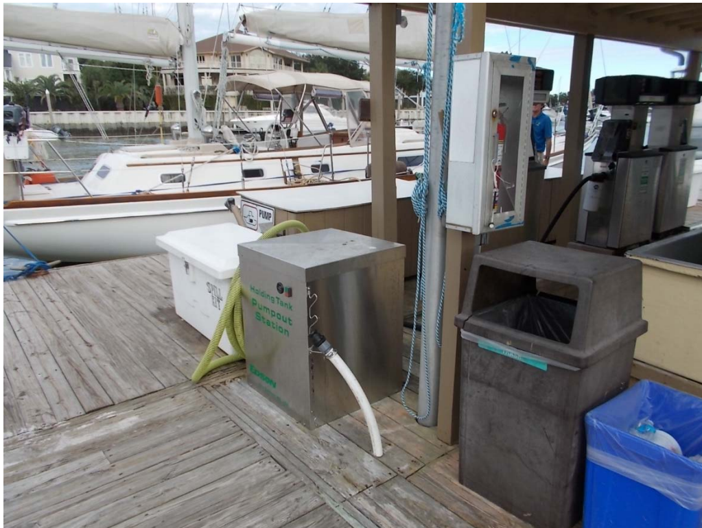
Existing, Fuel Dock
