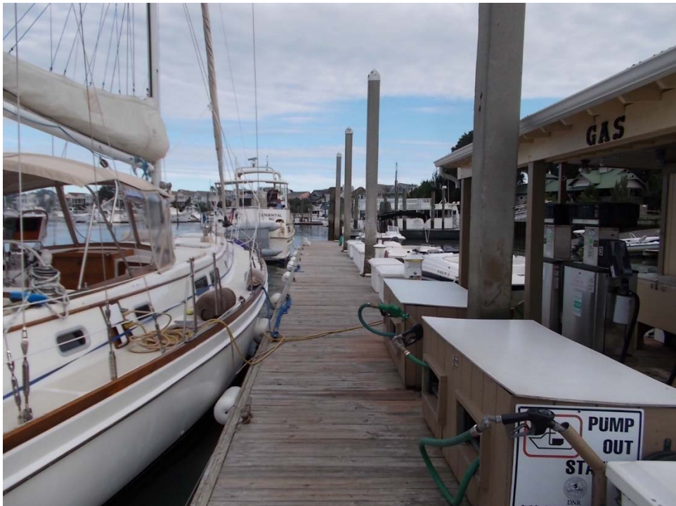
Existing Fuel Dock
