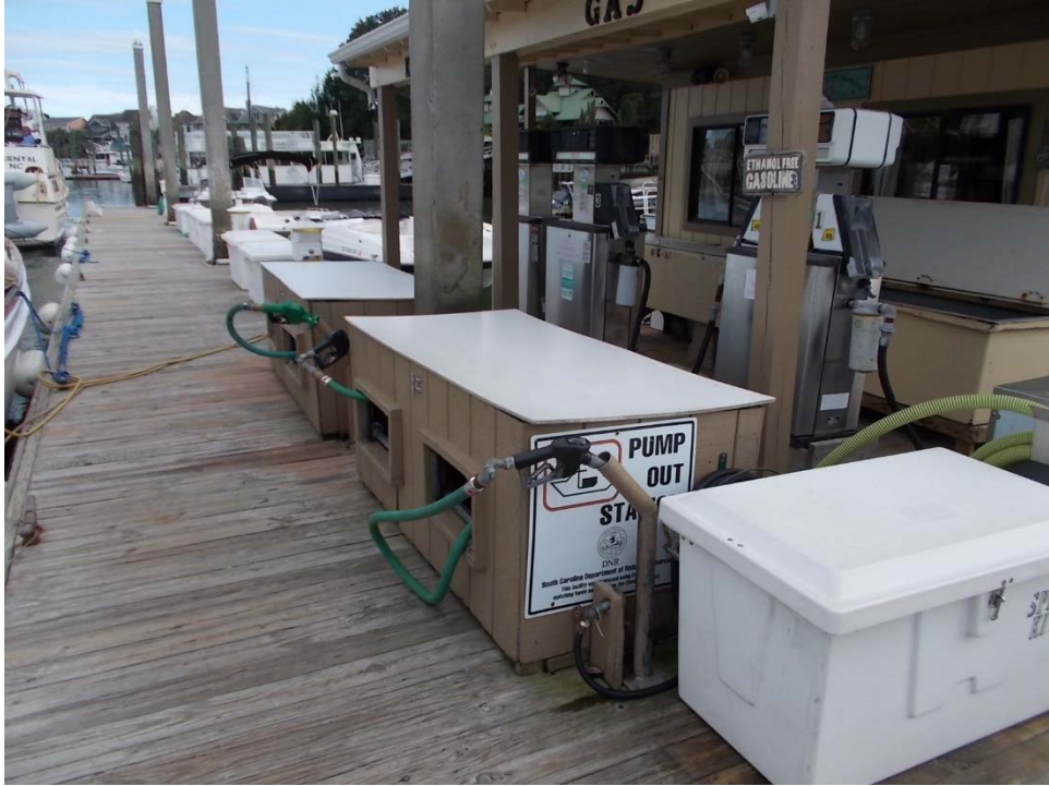
Existing Fuel Dock
