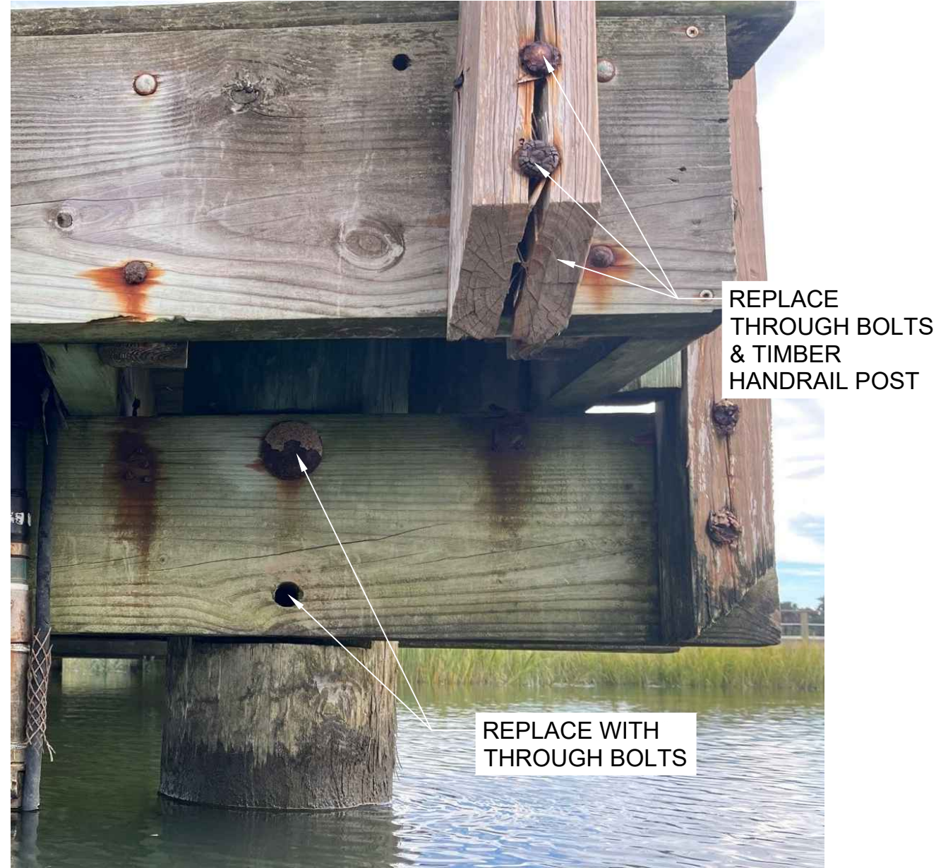
ACCESS PIER - HARD WARE AND HAND RAIL POST
