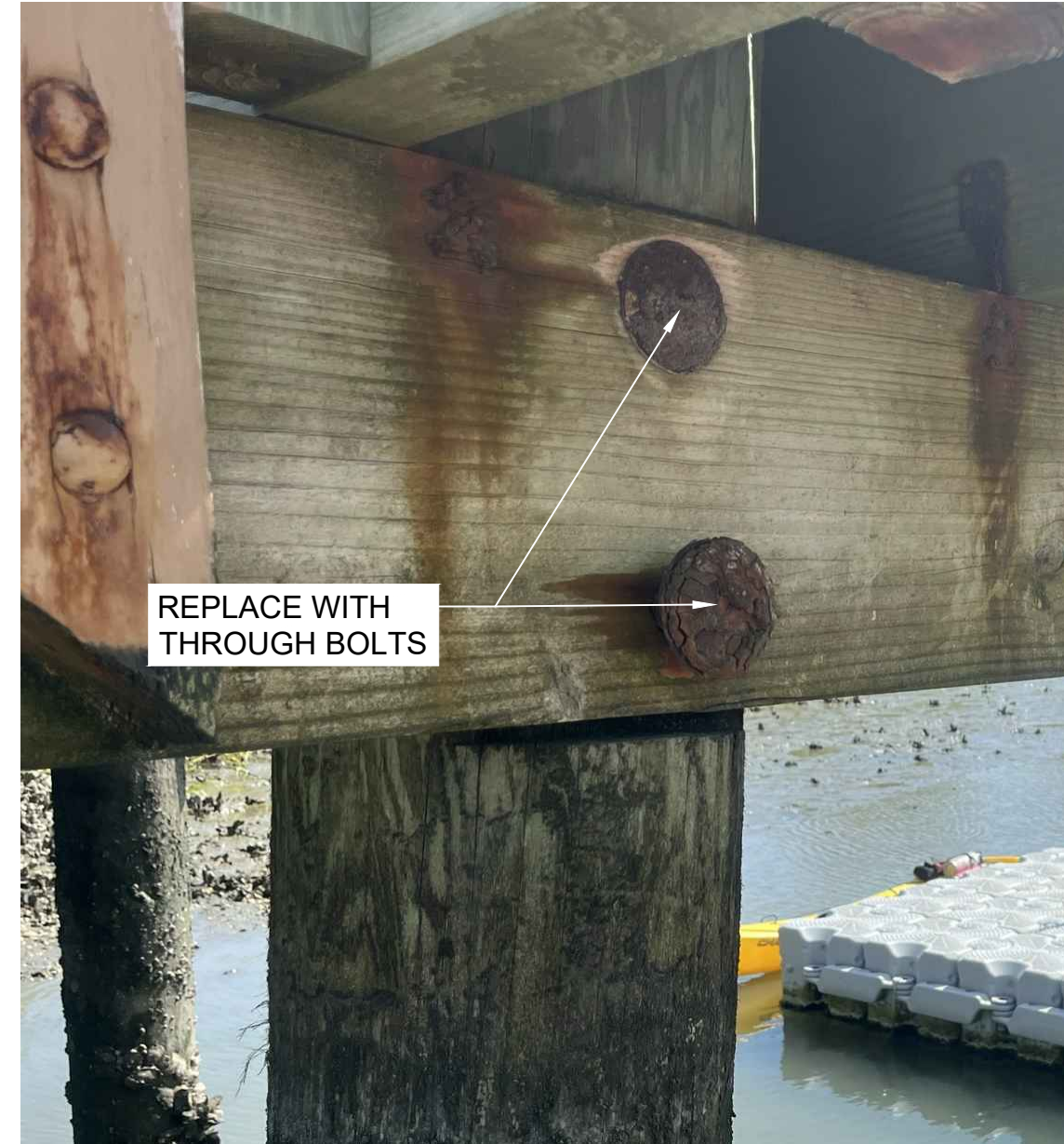
ACCESS PIER - HARD WARE AND HAND RAIL POST
