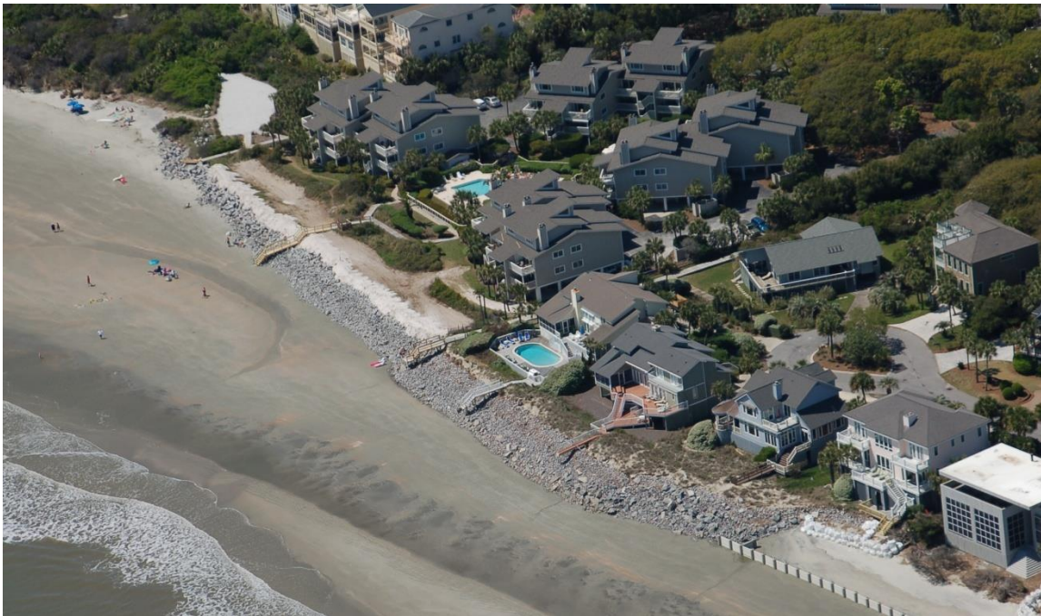
Figure 19. April 5, 2016 photo of exposed rock revetment near Seagrove/Beachwood East.
