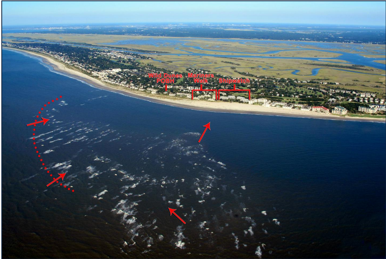
FIGURE 3.41. Aerial image of the migrating shoal offshore of northeast Isle of Palms. The general direction of sand movement is shown by the arrows. [Photo taken 25 September 2012 by SB Traynum]
