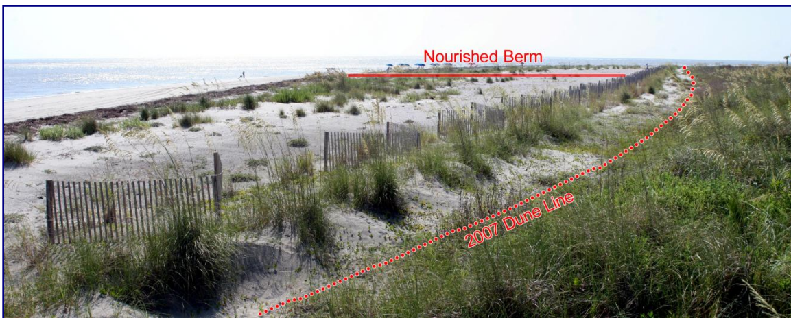
FIGURE 3.6. [UPPER] View inland of Reach 7 from the 17 th tee. [MIDDLE] View seaward of Reach 7 from the 17 th tee. [LOWER] View seaward of the nourished area of Reach 7. Vegetation has become well established seaward of the sand fencing. The pre-project dune line (red dotted line) is the dense vegetation ~25 ft to the right of the fencing in the image. [July 2012 –Photos by S Traynum]
