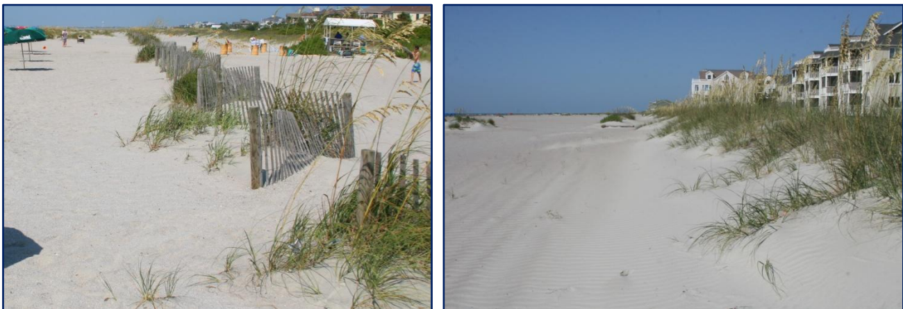
FIGURE 3.44. [LEFT] Sand fencing in Reach 5 in July 2012. There is less dune growth in this area than in Reach 6. [RIGHT] Sand fencing and vegetation in Reach 6 near Port O'Call in July 2012. [Photos by SB Traynum]
