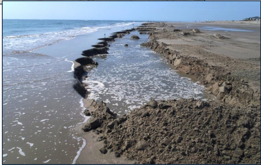
FIGURE 14. Construction photos of the project in March 2012.
