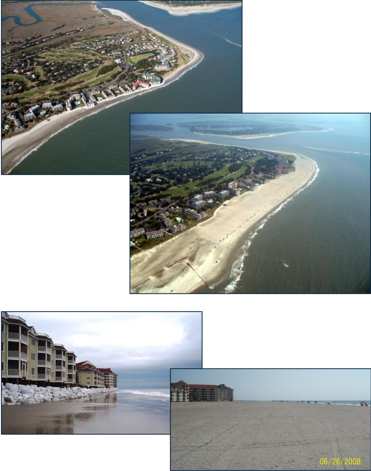
FIGURE 7. Aerial and ground photos of Reach B of the project area before (left images) and after (right images) nourishment. Over 550,000 cy of sand were added to the area, widening the beach by over 300 ft. The northern end of this reach has been an erosional hot spot since the project and is the general location of the current shoal-management project.
