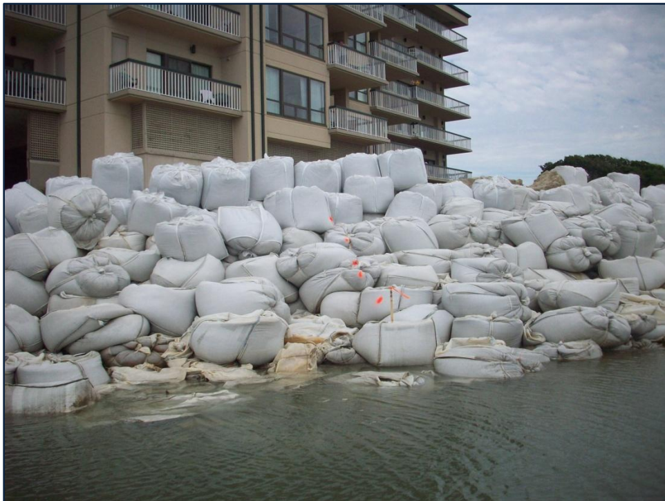
FIGURE 4. Small sandbags were placed in front of structures (upper); however, these quickly washed away, and large sandbags were placed on top of the remaining sandbags (lower). [Upper photo from Coastal Carolina University BERM Program]
