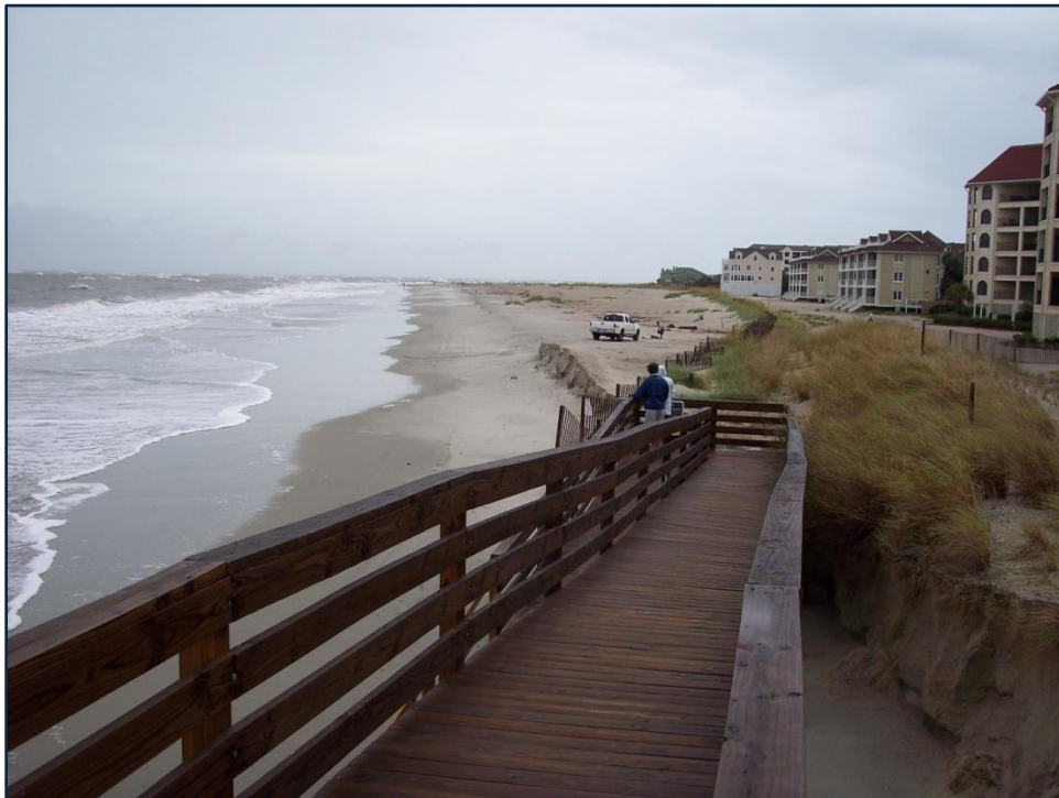
FIGURE 9. Condition of the shoal-management project fill area in August 2011 during Hurricane Irene , which passed offshore of South Carolina but produced significant wind and waves at Isle of Palms.
