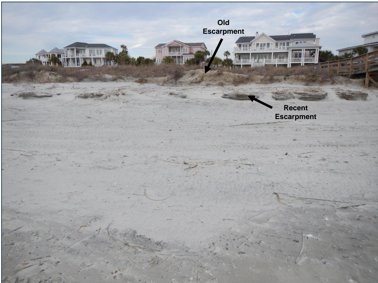
January 2014 image from station 4+00, looking landward. This area continues to rebuild following extensive erosion between 2011 and 2013. Note the older escarpment behind a more recent one, all fronted by a dry beach.
