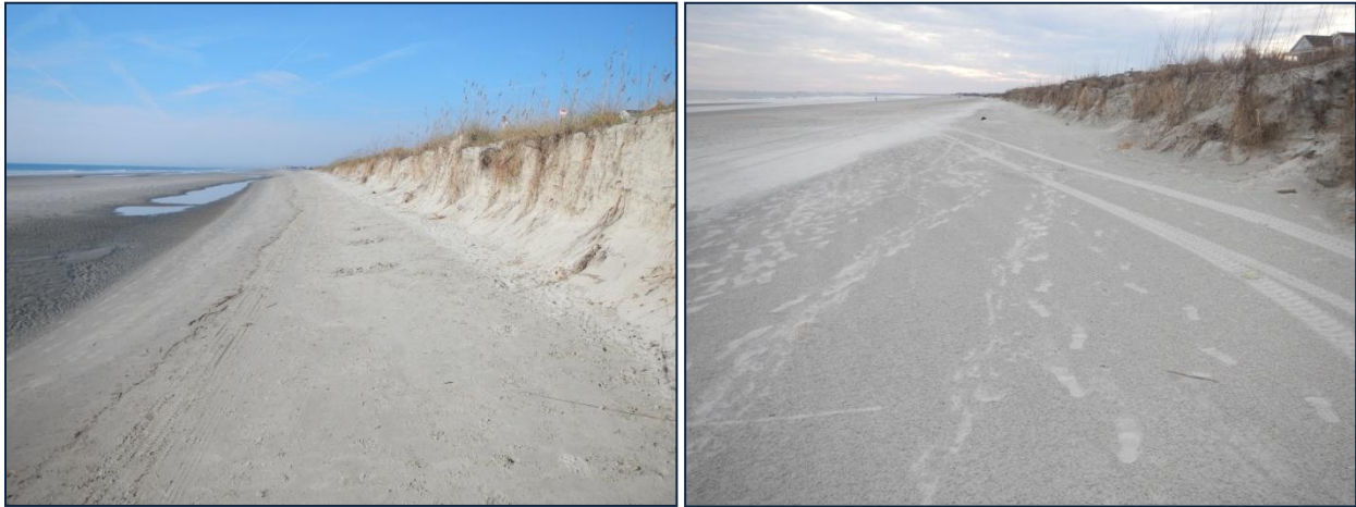
October 2013 (left) and January 2014 (right) images of station 50+00, looking west. This station gained 4.0 cy/ft between October and January, and the escarpment appears to be healing (note small buildup of sand at the base of the escarpment in the right image).
