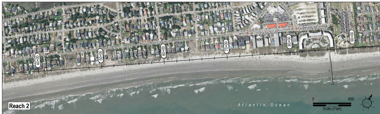
FIGURE 4.24. Baseline stationing along Reach 2 spanning between 6 th Avenue and the Sea Cabins Pier.
