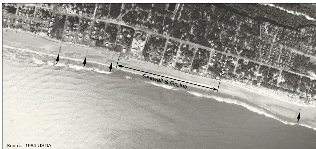
FIGURE 2.4. A seawall and groins were in place in 1984 between 46 th Ave to 53 rd Ave. Today, due to rapid accretion, these groins and seawalls have been buried.
