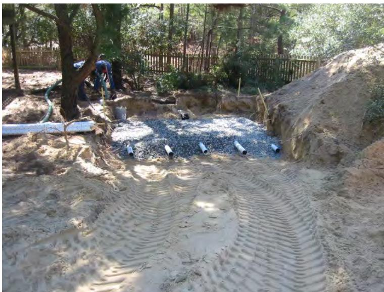
Figure 7-3. Septic system replacement
