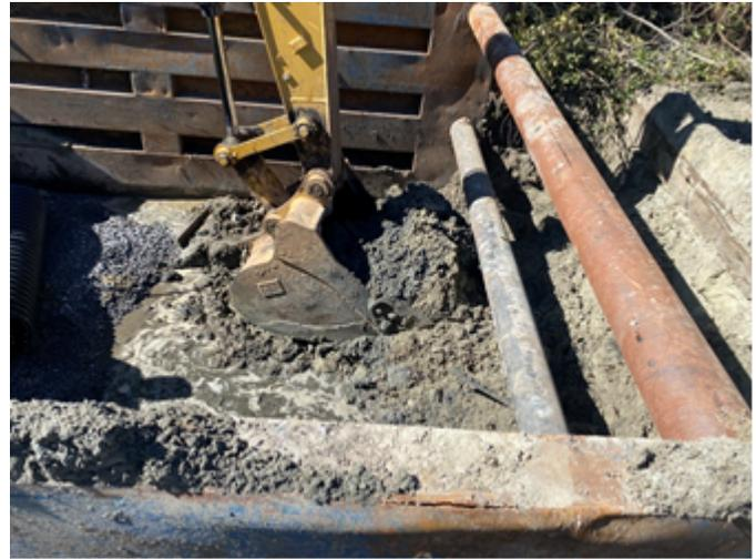
*Seewee Construction installing #57 stone and sump pumps to install pipes in wet soil conditions.*
